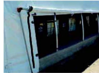
Adjustable roll-up sides move up and down to regulate air intake and exhaust, resulting in a premier environment.
