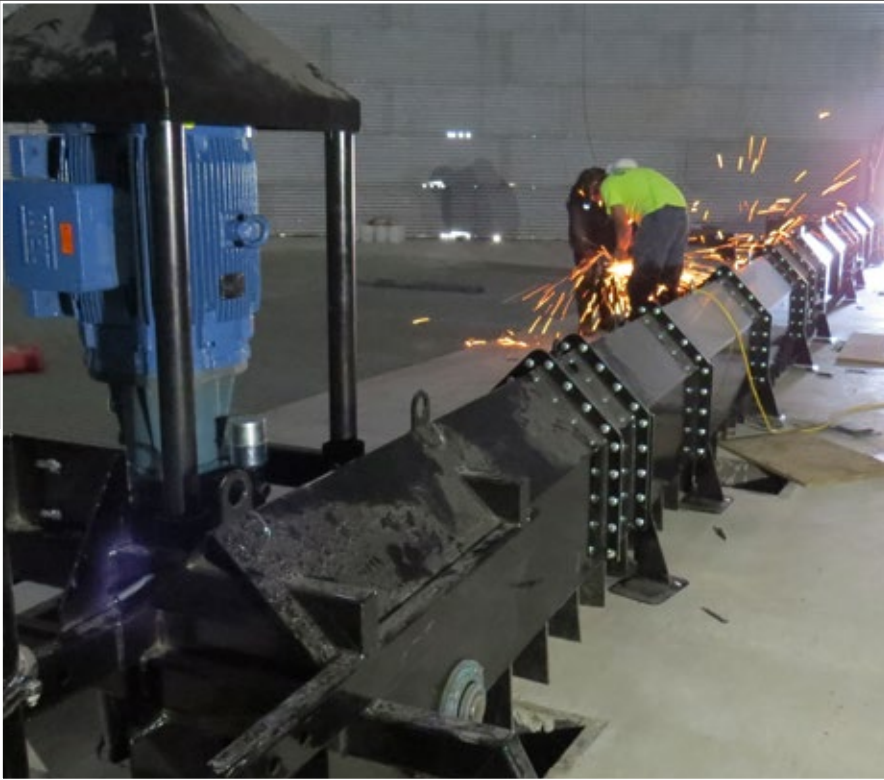
DPS 12K Sweep installation - AgWrx Coop, Aurora, SD
