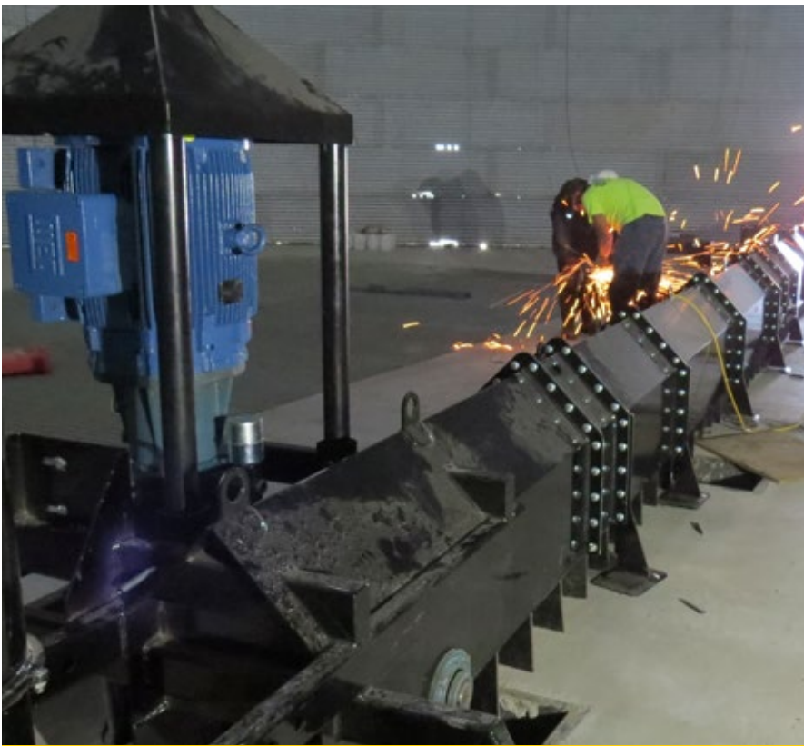
DPS 12K Sweep installation - AgWrx Coop, Aurora, SD
