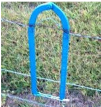
Step 4. Wrap spare wire around the stretched fence wire
