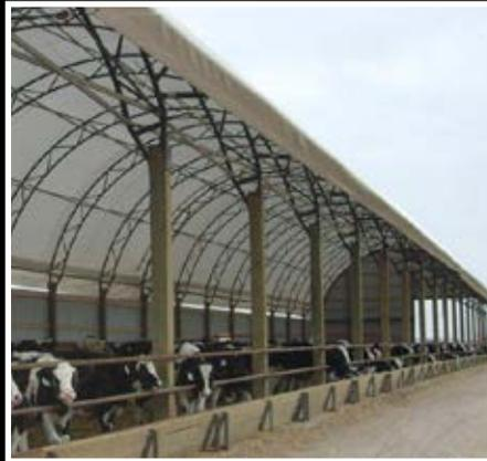
“The high roof of the building allows the system to rise up and out from the cattle so they don’t breath in all the moisture. And no poles down the center for free stall barns.”
