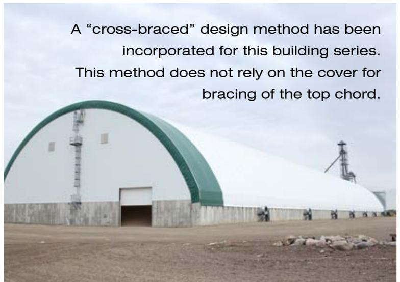
A "cross-braced" design method has been incorporated for this building series. This method does not rely on the cover for bracing of the top chord.
