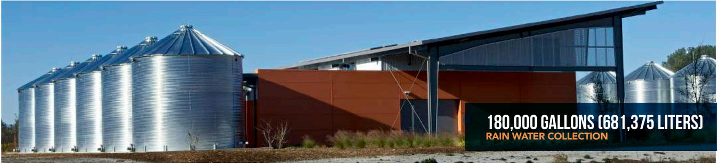
SCAFCO designs and manufactures water tank systems in various diameters with wall heights up to 14 feet (4.27 m) and capacities in excess of 100,000 gallons (395,000 Liters). (Larger tanks available upon request)
