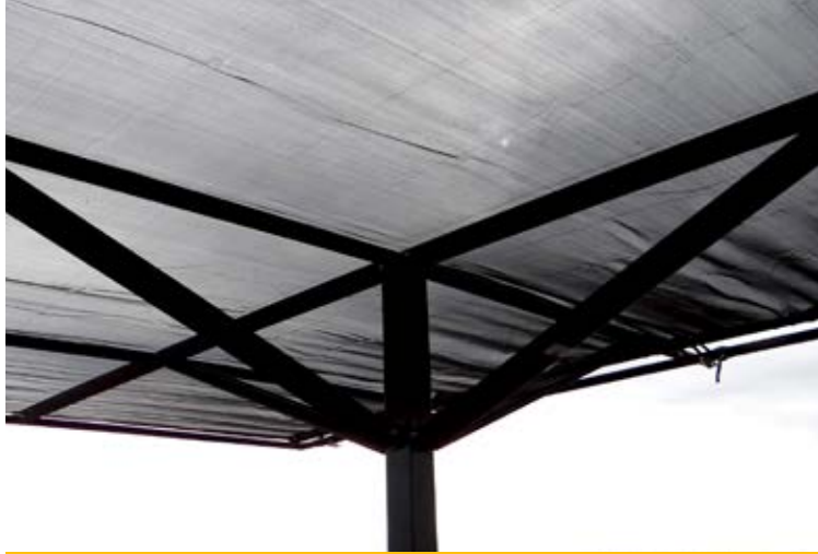
TWO 2.5" X 2.5" X 3/16" FORMED ANGLE BRACES
