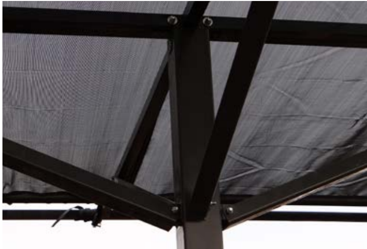
TWO 4.5" X 2.5" X 3/16" FORMED CHANNEL BRACES
